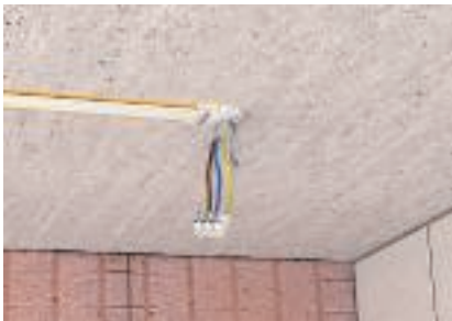
Impu-Fix adhesive application Ribbon conductors can be fastened with the Impu-Fix adhesive. Apply the adhesive to both sides with a brush and stick on the cable after drying. Fix the ribbon conductor using gentle knocks with a rubber mallet.
