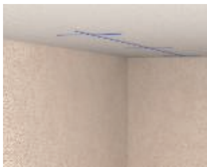
Mounting preparations Drawing of the exact position of the drill holes for the cable ties with a chalk line.
