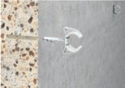
Snap clip application Draw the course and create the mounting holes.
