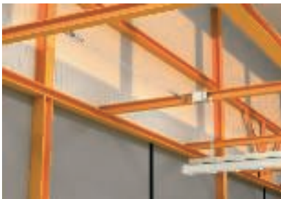
Steel wire tensioning cable systems Steel wire tensioning ropes can be used to support cable weights.
