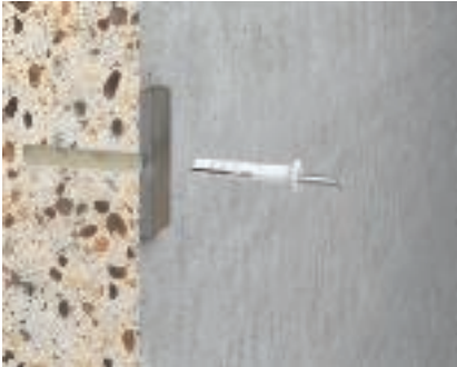
Knock-in anchor 910/SD application Push the knock-in anchor 910/SD through the fastening hole of the mounting hole and into the drill hole.
