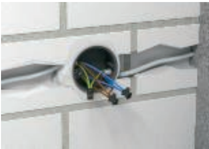
Application in a concealed distributor box With Dolü branch terminals (socket lamp-wire connectors), multiple cables can be screwed together in one terminal.
