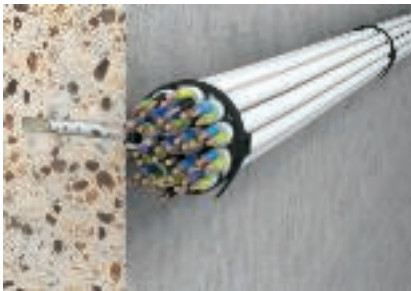
Complete installation, 910/STK I Fix the bundled cables in the drill hole with push-fit anchor.
