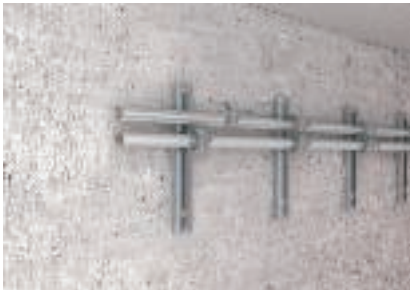
Wall mounting cables Cable mounting on profile rails with clamp clips.
