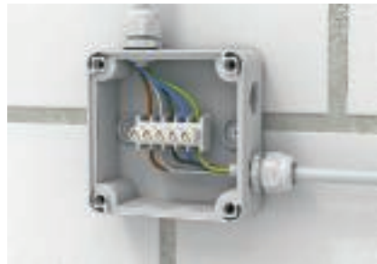
Earthing terminal There is the option of mounting an earthing terminal in the junction box.
