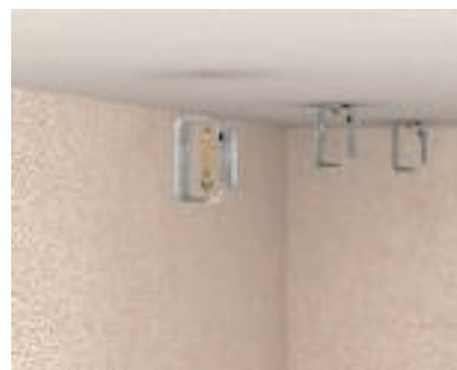
Ceiling mounting of the cable ties Simultaneous mounting of the cable ties with bolt ties as push-through mounting.
