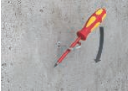
Ceiling hook application with multipurpose anchor Using a screwdriver, turn the hook into the anchor at least as far as the end of the thread.
