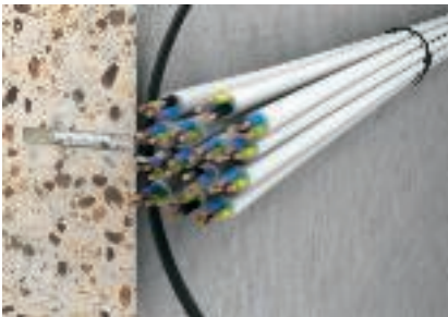
Fastening cables Tie cables to be installed together using the cable tie.
