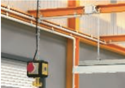
Cable fastening on suspended chain Cables can be fixed to and run on a chain using cable ties.
