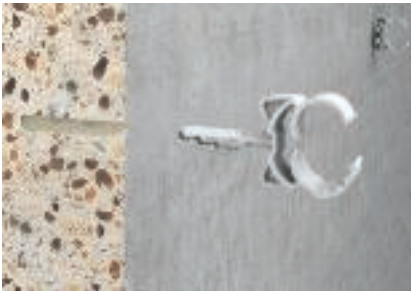
Click-snap clip application Draw on the exact position of the drill holes with a chalk line.
