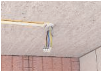
Terminal strip application For luminaire connection, wire ends can be secured with terminal clips.
