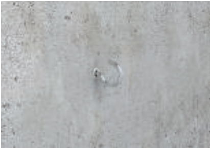
Ceiling hook application with multipurpose anchor The ceiling is now suitable to suspend luminaires using linked chains.
