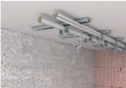
Ceiling mounting cables Cable mounting on profile rails with clamp clips.
