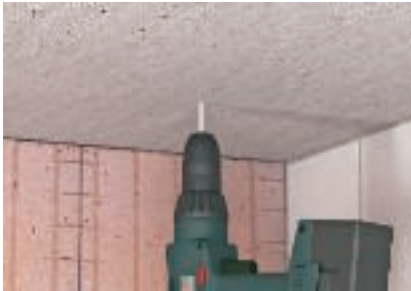
Bolt tie MMS-ST application Drill a hole with a diameter of 5 mm.
