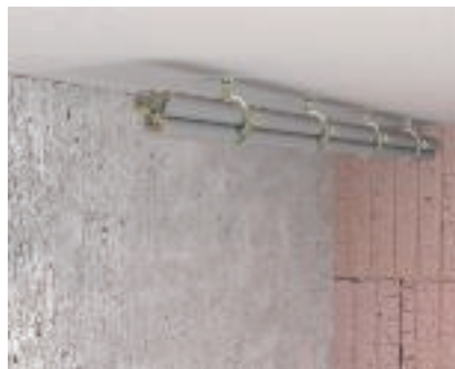
Ceiling mounting of cable bundle with spacer clip 732
