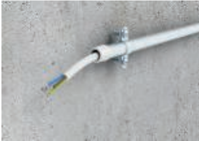
Pipe end socket application Now pull cables through the pipe.
