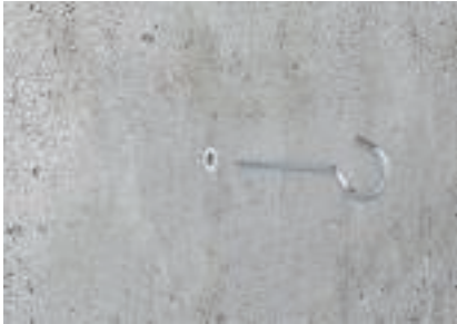
Ceiling hook application with multipurpose anchor Turn the ceiling hook into the anchor up to hand tightness.
