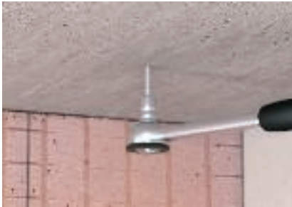
Bolt tie MMS-ST application Turn the tie in using a cordless screwdriver, drive screwdriver or by hand.
